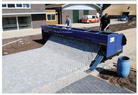
Figure 9. Bricklaying Machine
